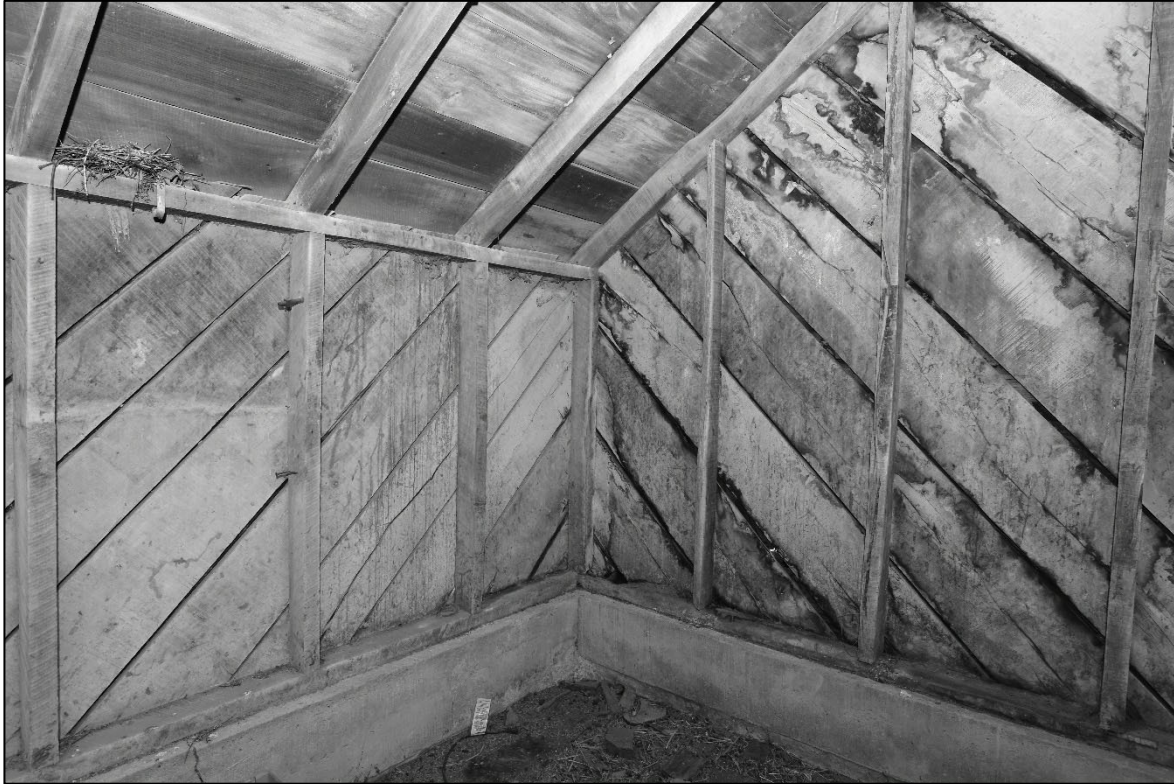
Photo 12. Detail of diagonal plank wall sheathing in northeast corner, looking northeast
