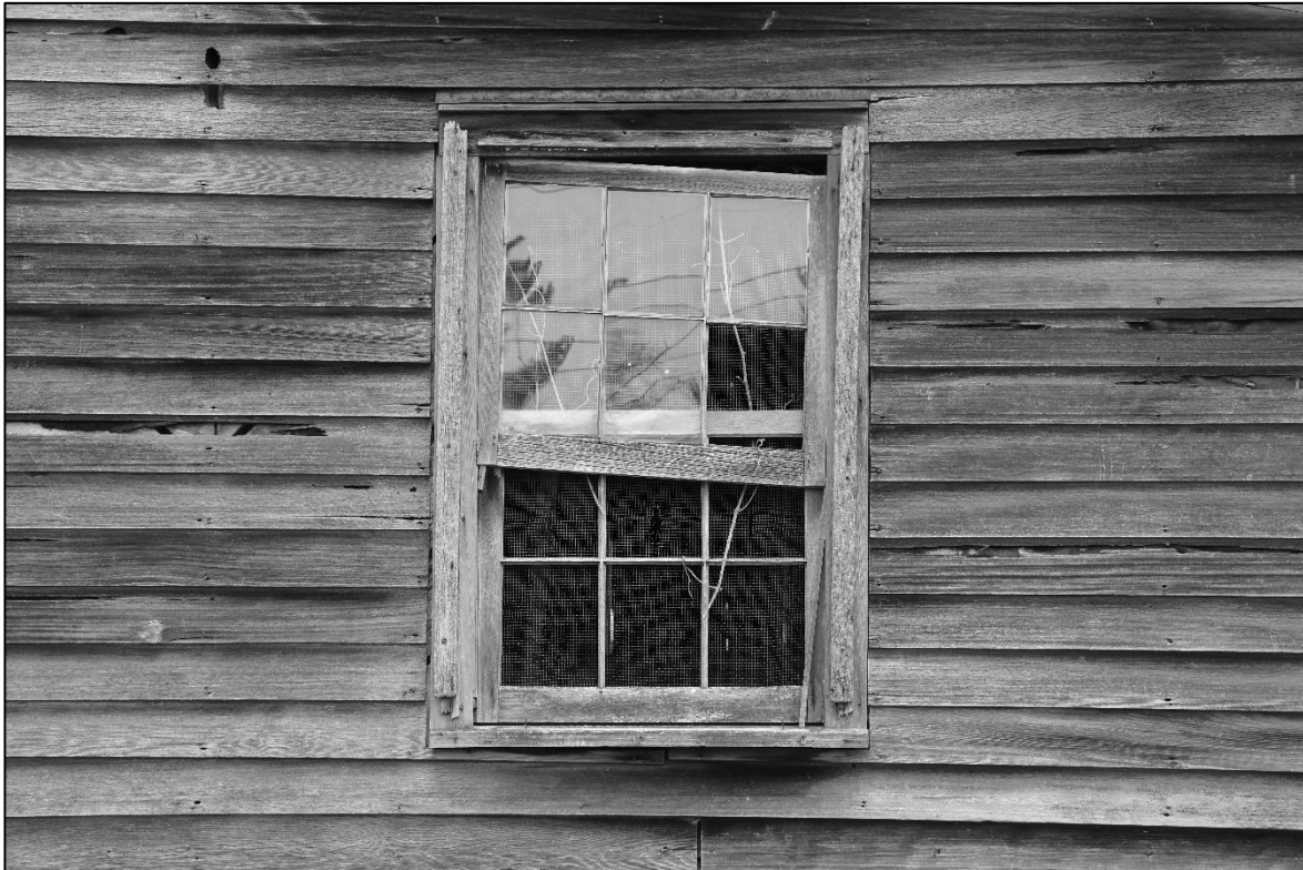
Photo 6. Detail of double hung window on west elevation, looking east
