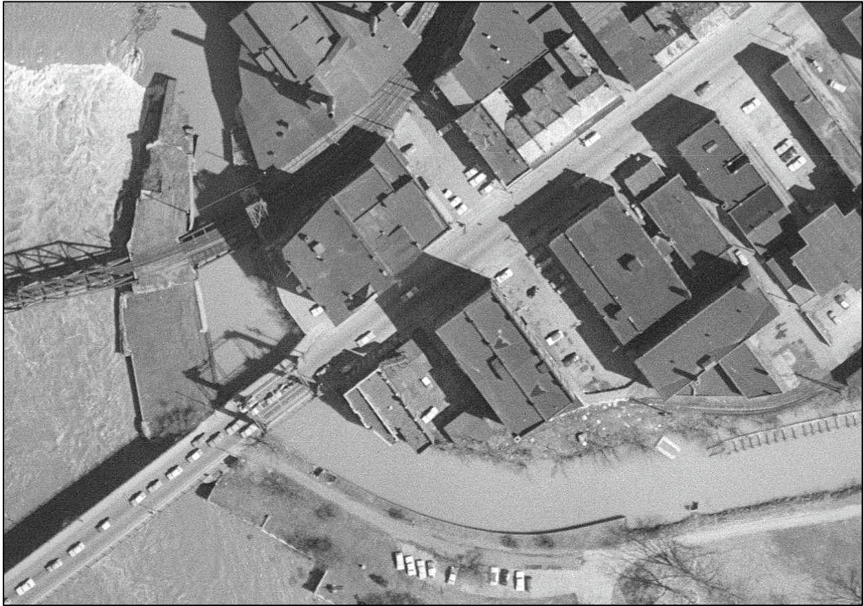
Figure 19. Detail from 1966 aerial photograph showing the original 1894 building and the 1913 addition in the center just north of the canal.
