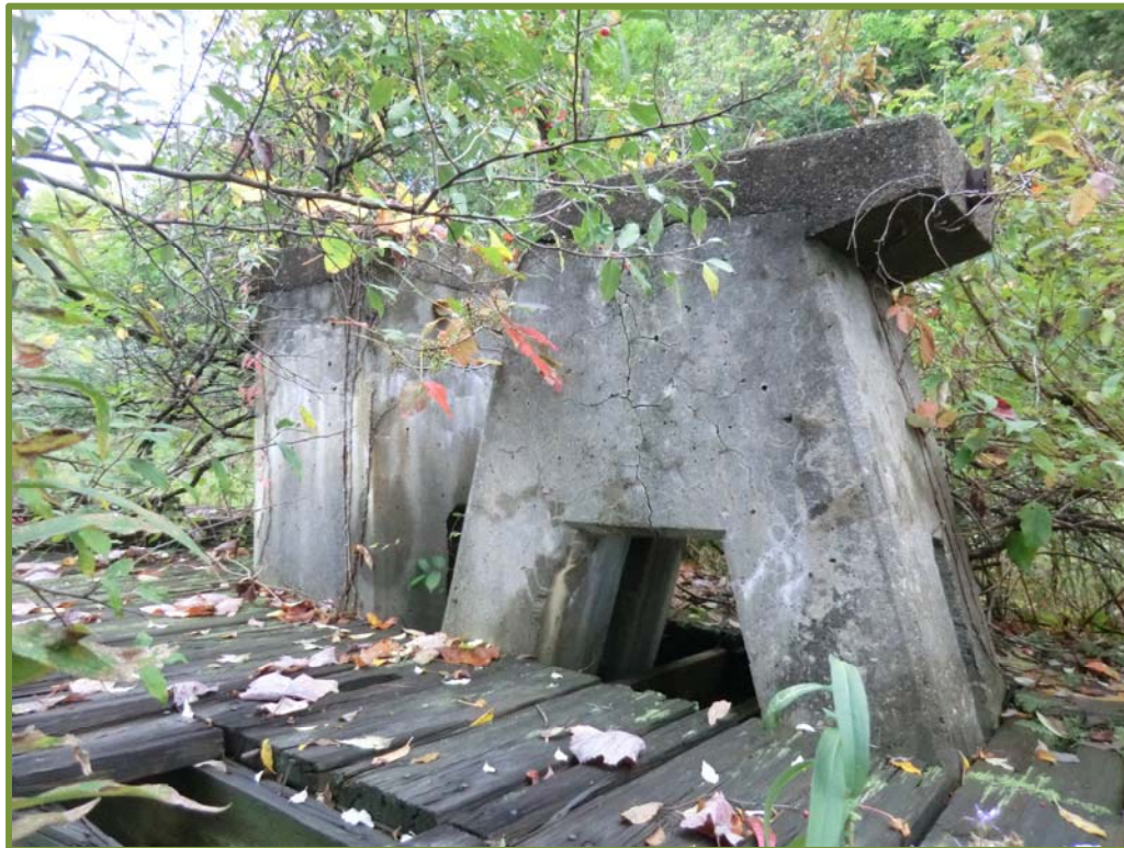
Photo 4. Detail of 0-m and 1-m pillars, looking east
