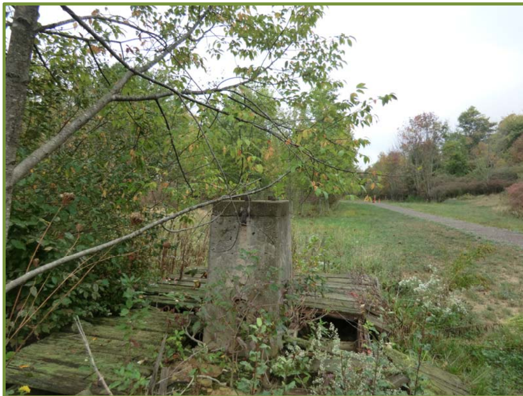
Photo 18. View over 250-m pillar toward 125-m pillar, looking southwest
