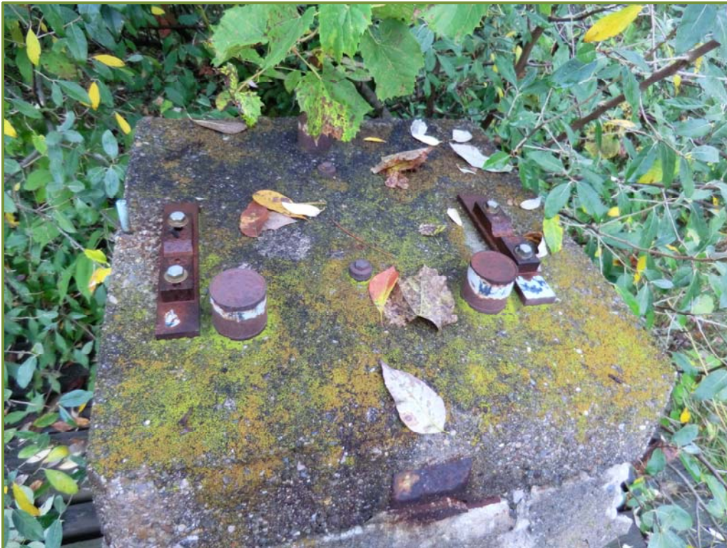
Photo 13. Detail of top of 25-m pillar, looking southeast
