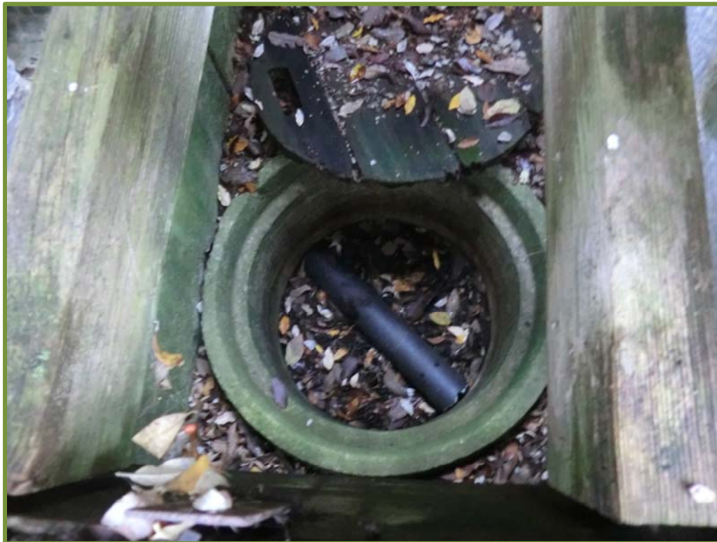
Photo 16. Detail of foundation of 125-m pillar, looking southeast
