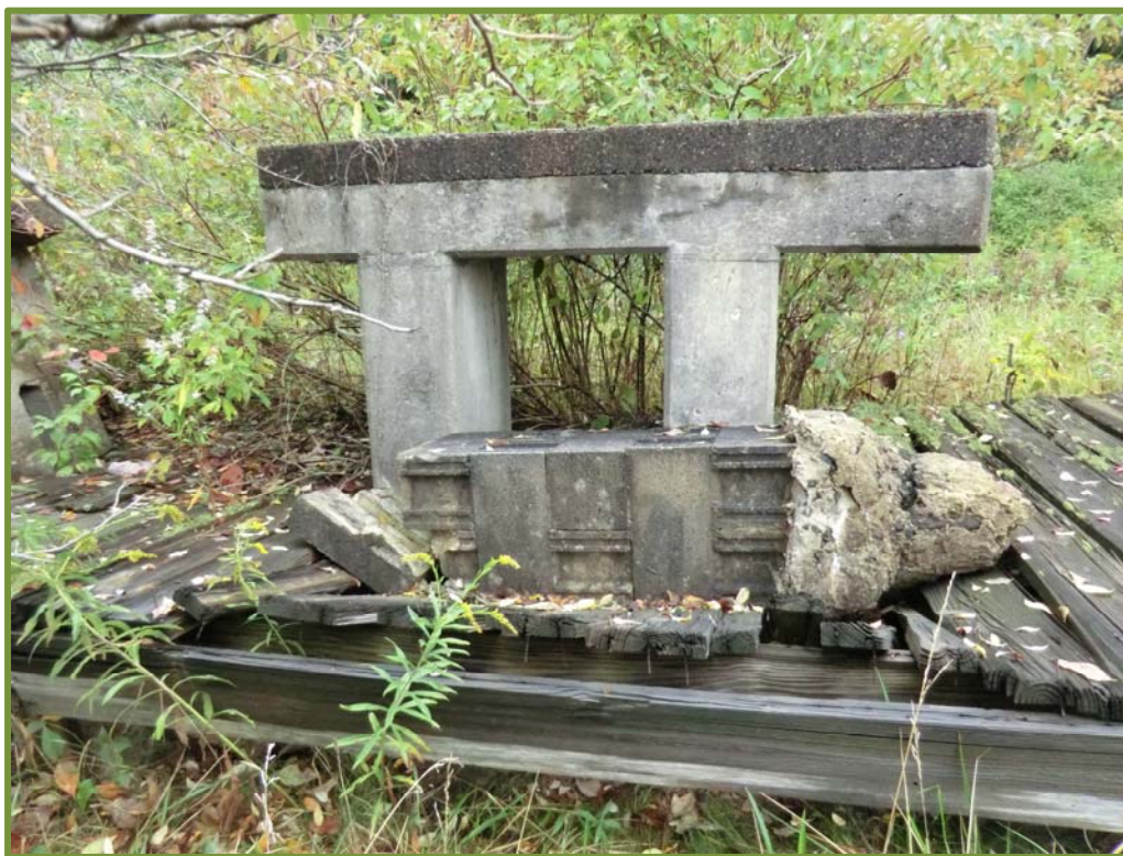
Photo 2. Detail of Comparator Stand including unrelated demolition debris, looking southeast
