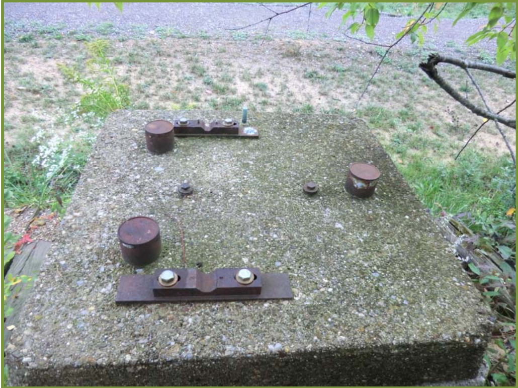
Photo 20. Detail of top of 250-m pillar, looking northwest
