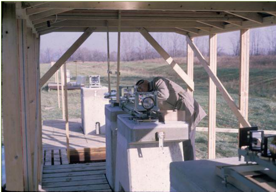
Figure 7. Ca. 1966 photograph showing detail of 0-m and 1-m pillars (photo courtesy of OSU Mansfield)
