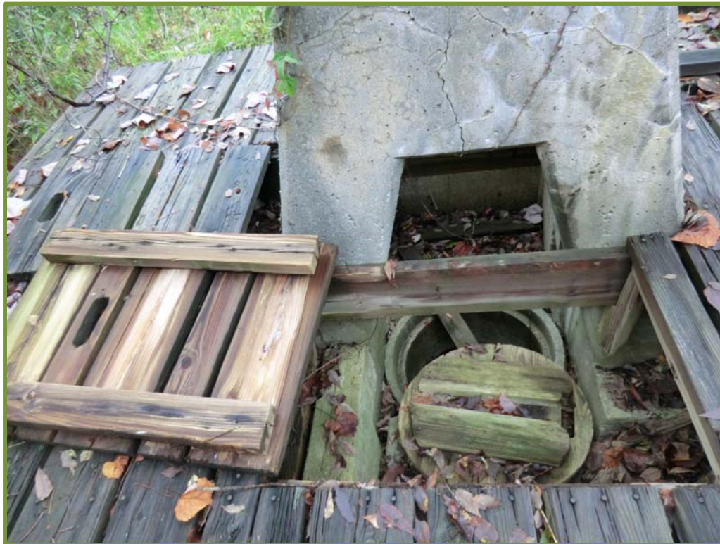
Photo 10. Detail of open trap door leading to base of 5-m pillar, looking northwest
