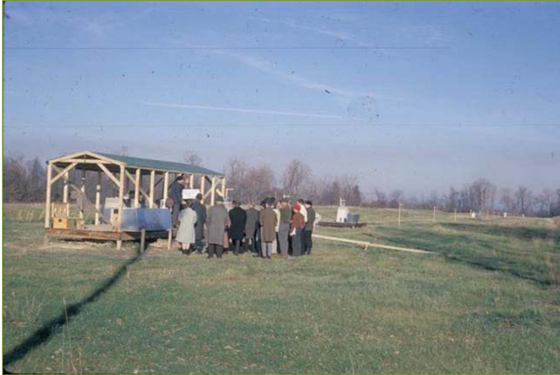
Figure 5. Ca. 1966 overview photograph of the OSB (photo courtesy of OSU Mansfield)
