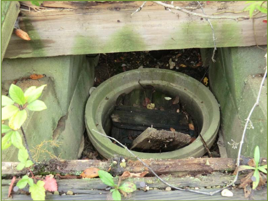
Photo 19. Detail of foundation of 250-m pillar, looking southeast
