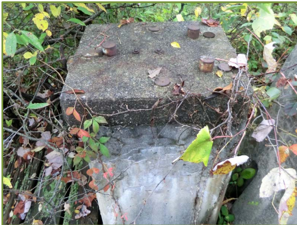
Photo 6. Detail of top of 5-m pillar, looking southeast
