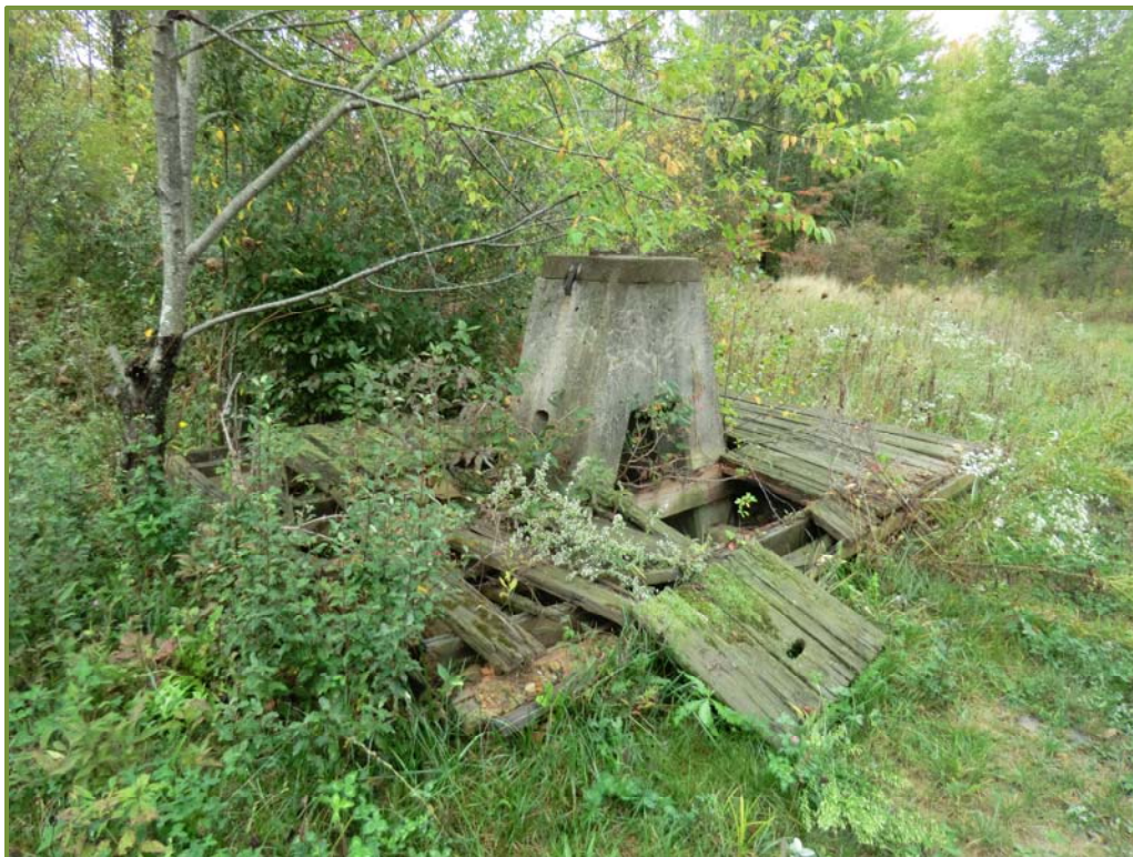
Photo 17. 250-m pillar, looking south
